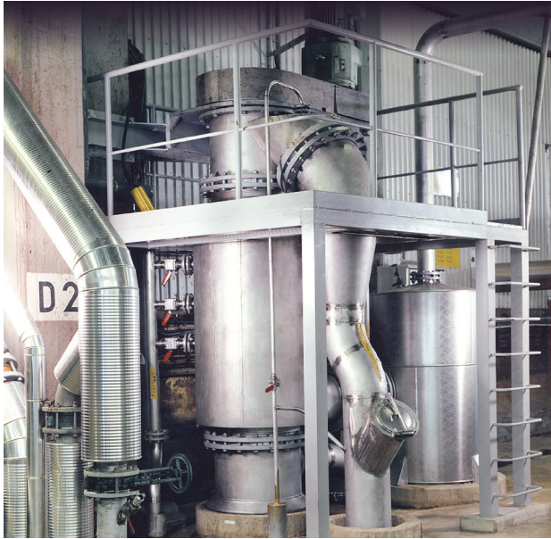
Raditrim-K secondary knotter screen installation
