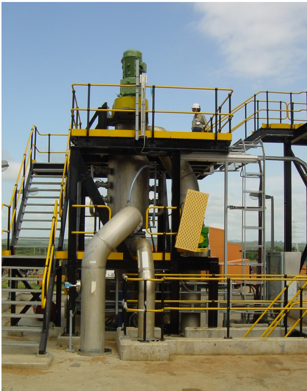
Raditrim-K secondary knotter screen installation
